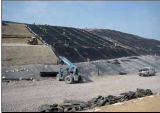
Workers unroll heavy plastic liner on the Cell 5 side slope, ultimately connecting the ‘panels’ both to each other and the bottom liner covering the soil berm. The rows of black strips on top of the soil (left side) are ‘geonet’ plastic barriers placed to protect sub-cap gas and leachate collectors.
