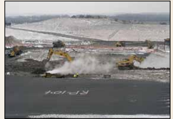
Workers start excavation of the 400,000 cubic yards of buried garbage between the expansion area and the original 88 acre footprint per the Settlement Agreement.
