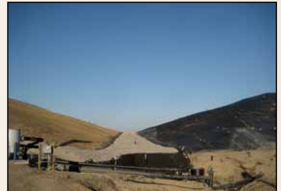
Isolation Break completed the bifurcation of the new expansion area from the existing 88 acre footprint. Left side of picture is the seeded northern expansion portion of the landfill. Right side of picture is the temporary capped existing 88 acres.
